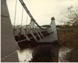
B1706 Wollaston Suspension Bridge Warrnambool
