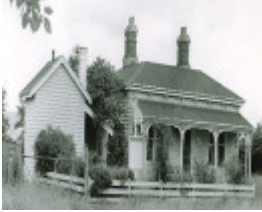
B2277 Old Police Buildings Covvarr
