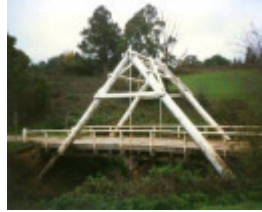
B6838 Hiawatha A Frame Bridge
