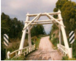
B6838 Hiawatha A Frame Bridge
