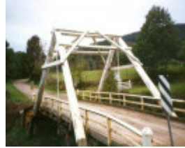
B6838 Hiawatha A Frame Bridge
