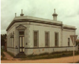
B0774 Fmr Bank Of Victoria Port Albert
