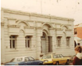
B4978 RSL Building
