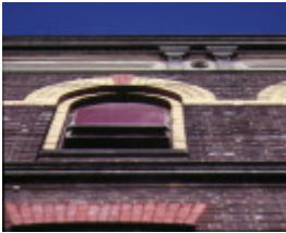
former denton hat mills nicholson street abbotsford detail of window
