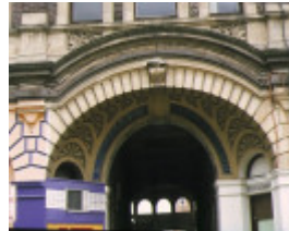
former mining exchange ballarat detail from front entrance oct1980
