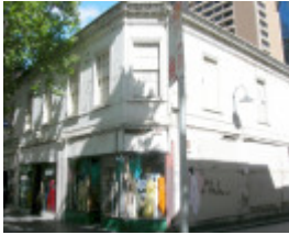
JOBS WAREHOUSE SOHE 2008
