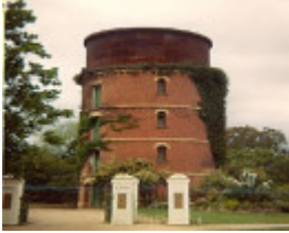
B4810 Brick Water Tower
