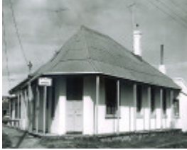
B1219 Fmr Derwent Hotel Wharf St Port Albert
