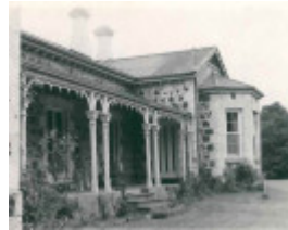
B2847 Benyeo Homestead Side View
