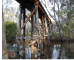
B6921 Fulham Rail bridge
