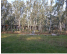
B6921 Fulham Rail Bridge
