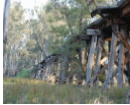
B6921 Fulham Rail Bridge
