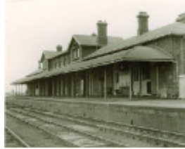
B2371 Railway Station Serviceton
