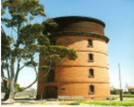
B2728 Water Tower Murtoa
