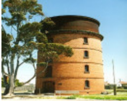
B2728 Water Tower Murtoa
