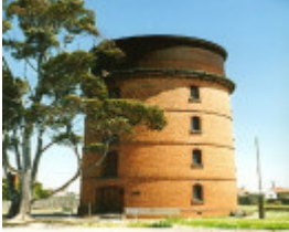
B2728 Water Tower Murtoa
