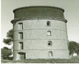
B2558 Water Tower
