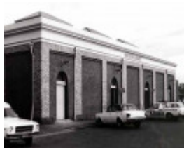
B3215 Railway Buildings
