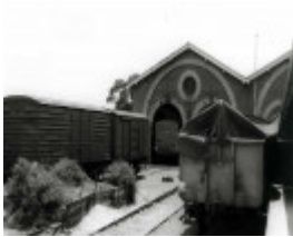
B3215 Railway Buildings
