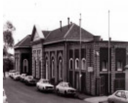
B3215 Railway Buildings
