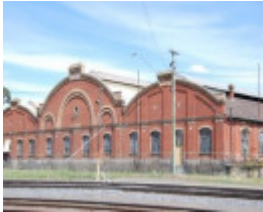
B3215 Railway Buildings
