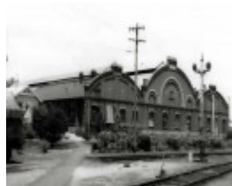
B3215 Railway Buildings
