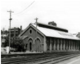
B3215 Railway Buildings
