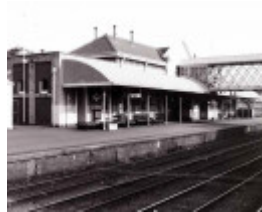
B3215 Railway Buildings
