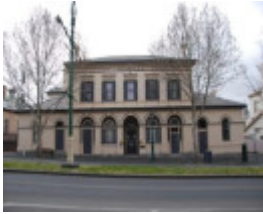
B1368 Sandhurst Trustees Co former Post and Telegraph Office
