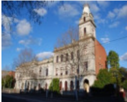
B5052 School of Mines Building - Group Classification
