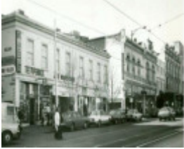
B7231 Bourke St East
