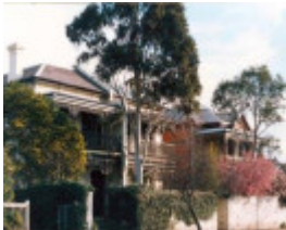
B7237 Hawthorn Grove Historic Precinct
