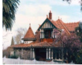
B7237 Hawthorn Grove Historic Precinct
