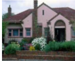
B7247 Beauville Ave Murrumbeena
