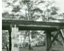
L10003 Rail Bridge Central Park
