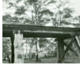
L10003 Rail Bridge Central Park
