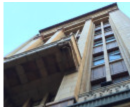
FORMER BANK OF NEW SOUTH WALES July 2016
