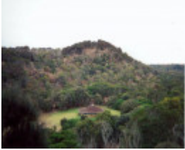
L10159 Tower Hill Information Centre
