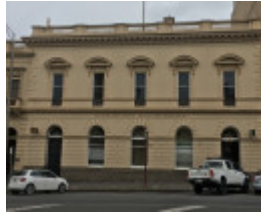
Former Bank of NSW 2
