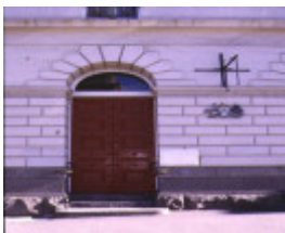
bank of nsw ballarat detail south external door
