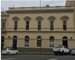
Former Bank of NSW 3
