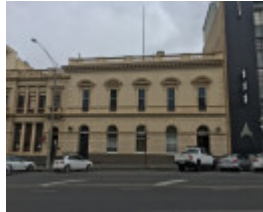
Former Bank of NSW
