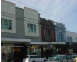
B7266 Kings Buildings, Burke Road
