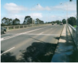
B7305 Barwon Bridge
