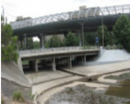
B7312 Flemington Bridge
