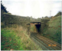
B7319 Harper's Lane Bridge
