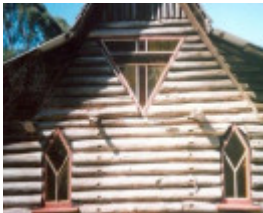
B7317 Log Church Rear Windows
