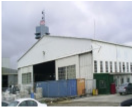
B7360 Fmr Comm Aircraft Hangar Site
