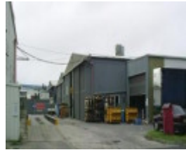
B7360 Fmr Comm Aircraft Hangar Site
