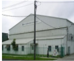
B7360 Fmr Comm Aircraft Hangar Site
