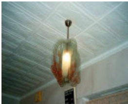
B7344 Lobby Ceiling
