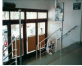
B7344 Entry Stairs
