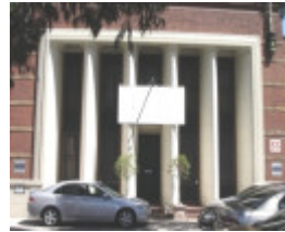
B7362 Fmr Drill Hall
