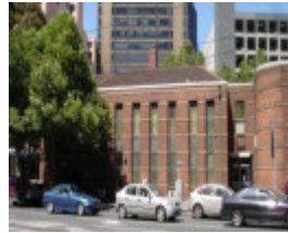
B7362 Fmr Drill Hall
