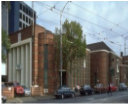
B7362 Fmr Drill Hall
