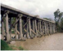
B7371 Latrobe River Bridge
