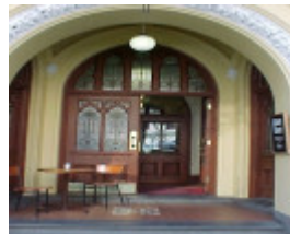
professional chambers collins street melbourne entrance detail sep1999
