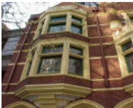
professional chambers collins street melbourne window detail sep1999
