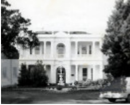
B1533 Armadale 461 St Kilda Rd Melbourne
