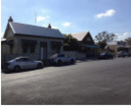
Falls Road Precinct
