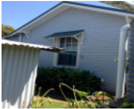
South gable window, 425 Harding-Lawson Rd
