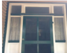
Front entrance door, 14 Bridge St
