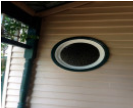
Porthole window, 14 Bridge St
