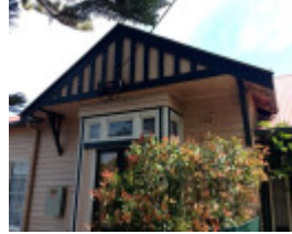
'Flying' gable, 14 Bridge St
