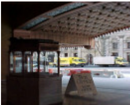
regent theatre collins street verandah detail jul1999
