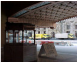
regent theatre collins street verandah detail jul1999
