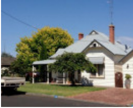
House, 42 Brown St
