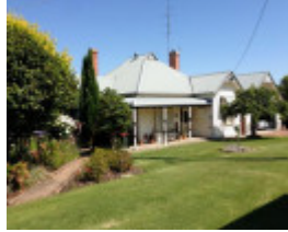
House, 42 Brown St
