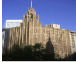
1 manchester unity building collins street melbourne front elevation feb1986
