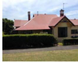
House, 19 Long St
