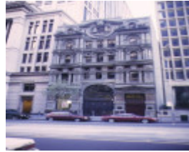
1 mercantile bank collins street melbourne front view
