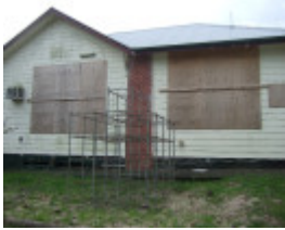
Bena School (former)
