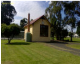
Port Franklin State School No.4280 (former)
