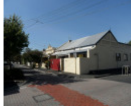
57-63 Stafford Street, looking east
