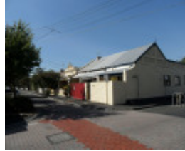
57-63 Stafford Street, looking east
