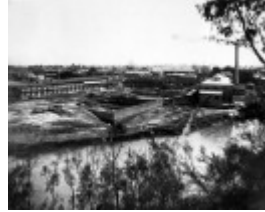
1918 - Yarra Falls construction.jpg
