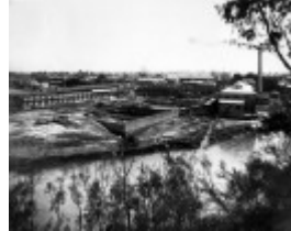
1918 - Yarra Falls construction.jpg
