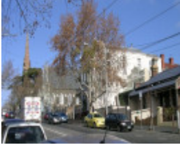
Church Street Precinct.JPG
