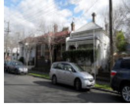
Late Victorian and Federation houses at 32-36 Charles St (recommended for inclusion in HO319)
